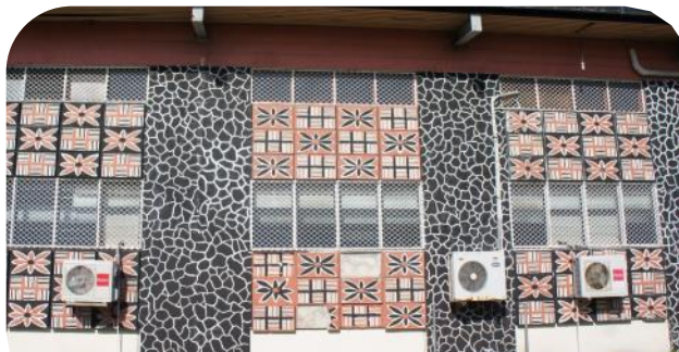
Fig. B1.5 Samoan patterns and materials on building façade
