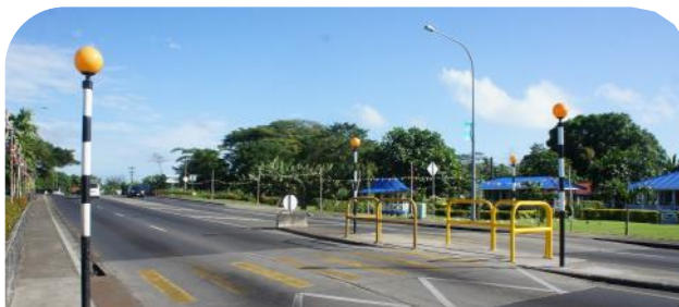
Fig. E3.2 Pedestrian crossing with raised hump, pedestrian refuge area and flashing lights
