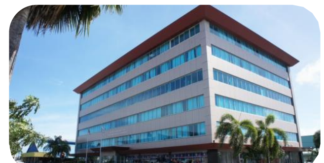
Fig. D1.2 Existing taller building in Apia waterfront area
