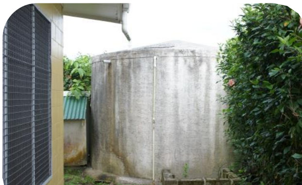
Fig. C8.1 Stormwater detention tank
