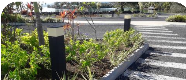
Fig. C5.1 Bollard lights provide better illumination for pedestrians than tall lighting poles designed for vehicles
