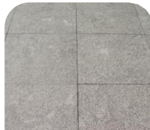
Fig. C7.2 Non-slip slate tiles
