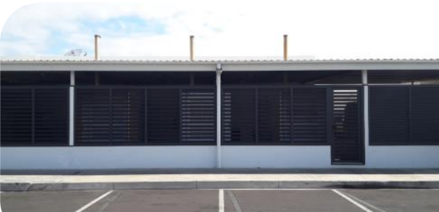
Fig. D7.1 Screen air-conditioning units from public view
