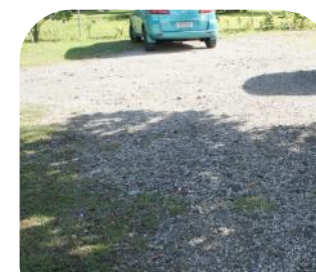
Fig. C2.2 Gravel parking area allows infiltration of rainwater
