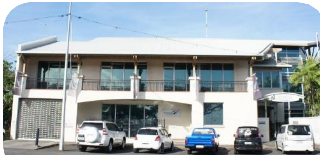
Fig. D7.2 Service piping (downpipes) are integrated into this building design
