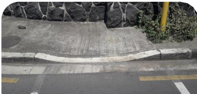
Fig. E3.1 Example of kerb ramp
