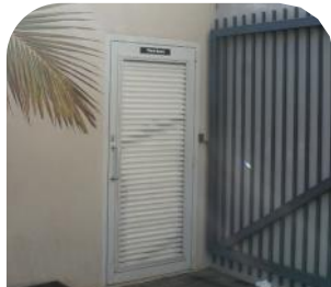
Fig. C6.2 Clear access to service entrances
