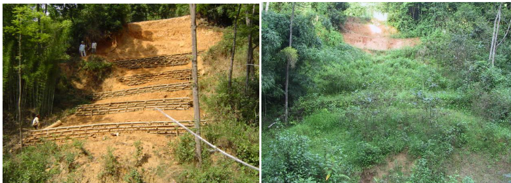
Figure 11. Bamboo crib wall on experimental site 3 in Badikhel/Lalipur, Nepal, on May 2004 (left) and October 2005 (right).
