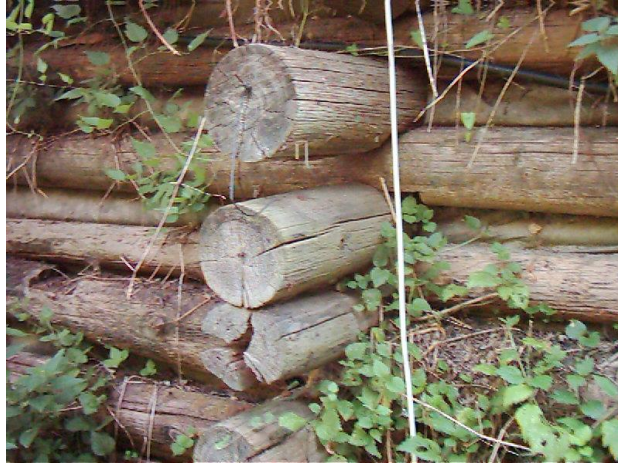
Figure 8. The condition of wooden crib wall (constructed almost vertical) after 20 years of the construction, in Königstätten, Lower Austria (July, 2007).
