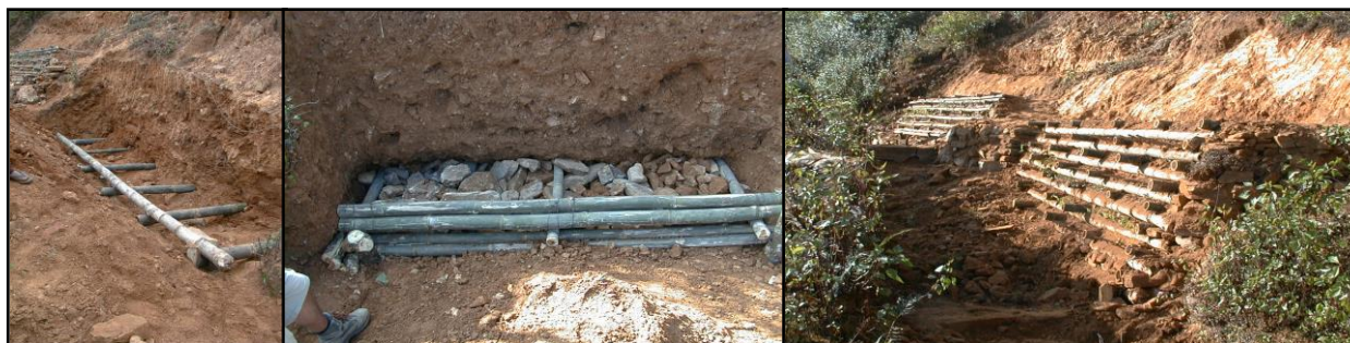
Figure 7. Bamboo crib wall construction stages.
