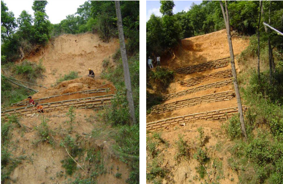
Figure 3. View of project site B (landslide before and after construction of bamboo crib wall), Badikhel/Lalitpur, Nepal (May, 2004).
