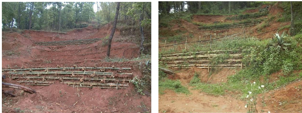
Figure 9. Bamboo crib wall on experimental site 1 in Badikhel/Lalipur, Nepal, on May 2003 (left) and on August 2003 (right), (Tardio et al., 2018).
