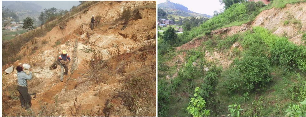
Figure 10. Bamboo crib wall on experimental site 2 in Badikhel/Lalipur, Nepal, on December 2003(left) and October 2005 (right)
