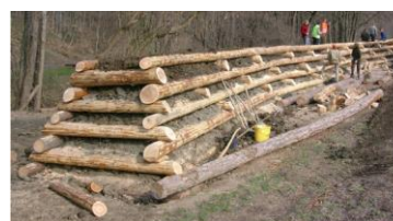
Figure 5. An example of wooden crib wall.
