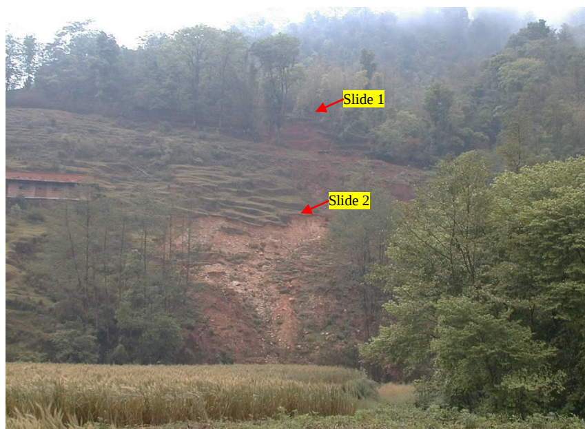
Figure 2. View of landslides at project site A in Badikhel/Lalitpur, Nepal (April 2003).
